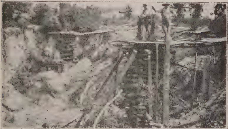
(26) A method in removing caved ground, at Susie Beeler mine.
